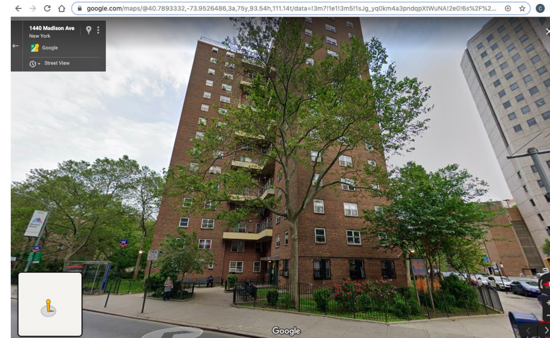
Public Housing Building - Hotspot #4
